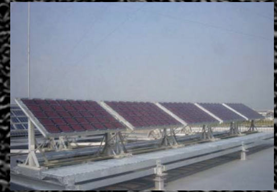
Kariya City at lat. 35°10'N, Azimuthal angle: 0° Facing due south, Tilted at 30°
